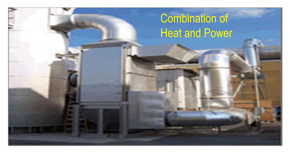
Energy in engine exhaust gas and engine jacket water can be recovered for heating or chilling application
